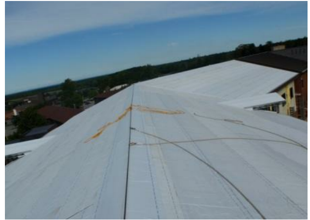
MFM Wind & Water Seal Installed on Air Force Base Roof
