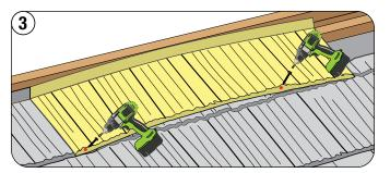
Install ridge cut panel across the ridge, aligning with the panel below. Fasten left end, then right end of the panel.
